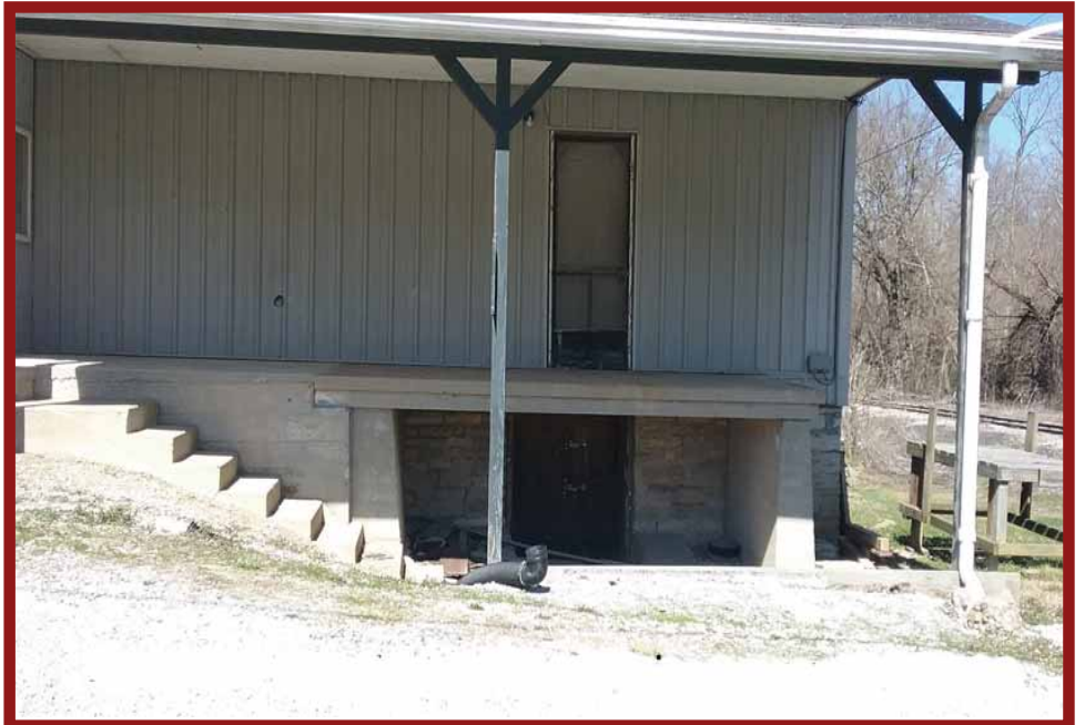
Basement of the Faikert Building, showing stonework from 1883.
