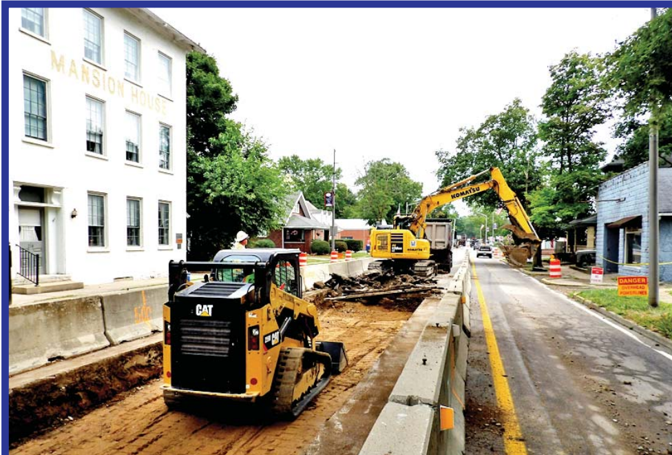
Milestone Contractors removing the interurban track in front of the Mansion House an early 1800 Inn still can be visited and enjoyed today. (Author Photo)
