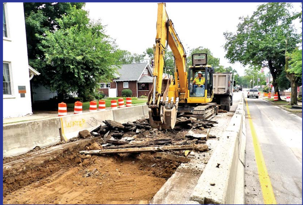
As the crew moves west along U.S. 40 the Milestone Contractors steadily remove track and debris replacing it with a smooth new pavement complete with center line . (Author Photo)
