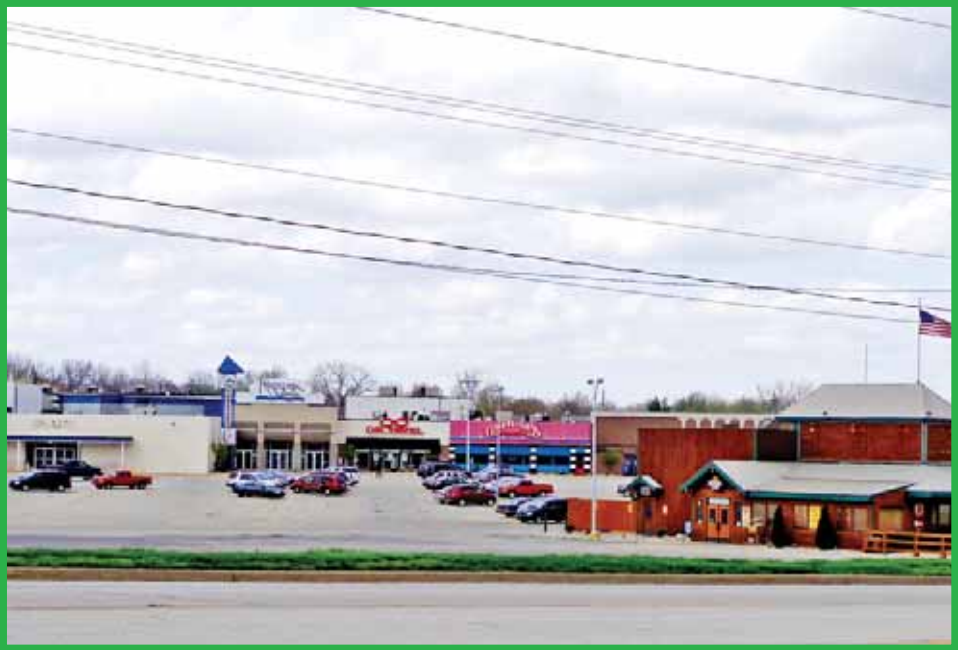
This photo taken from the east side of Scatterfield Road shows the Mounds Mall in the background and the Texas Roadhouse restaurant in the foreground. Both will be under water.
